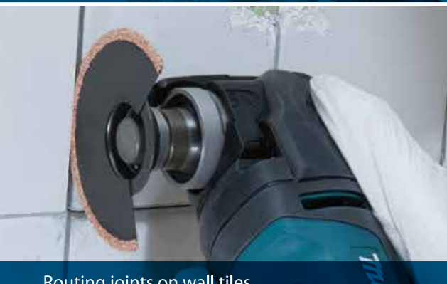
Routing joints on wall tiles
