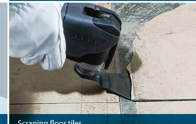
Scraping floor tiles
