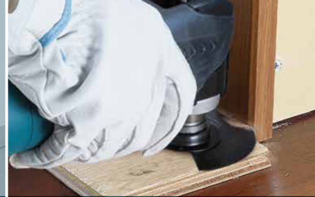
Wood flush cutting
