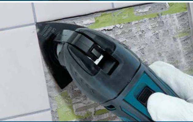
Removing mortar, tile adhesive
