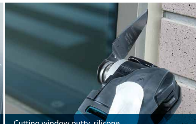
Cutting window putty, silicone
